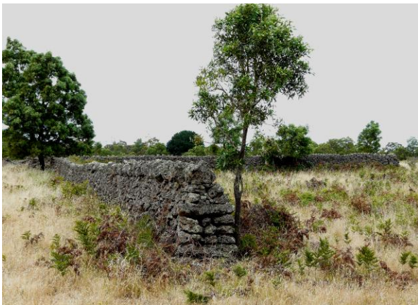
Photo 38 (above) – a drystone fence built in the volcanic landscape north of Lake Condah. Black Wattles have colonized the cleared area in this scene (Photo Dec. 2008).
