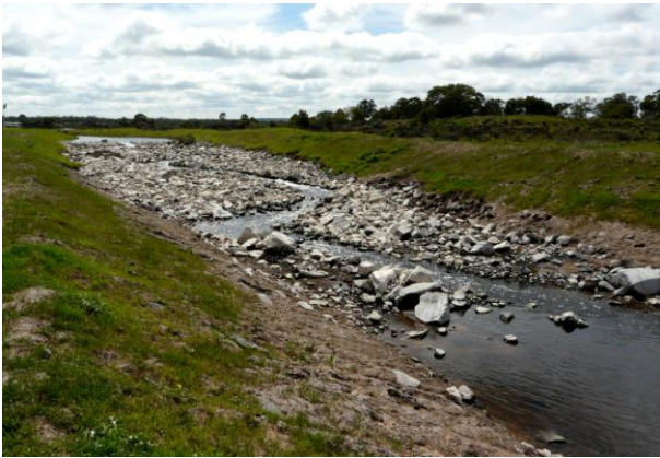
Photo 79 (above) – Lake Condah outlet weir and fish ramp built on Condah drain in April 2010 (Photo Oct. 2010).
