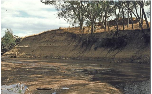
Photo 74 (above) – ‘improved’ Glenelg with eroded banks and trees about to fall into the stream (Feb. 1977).
